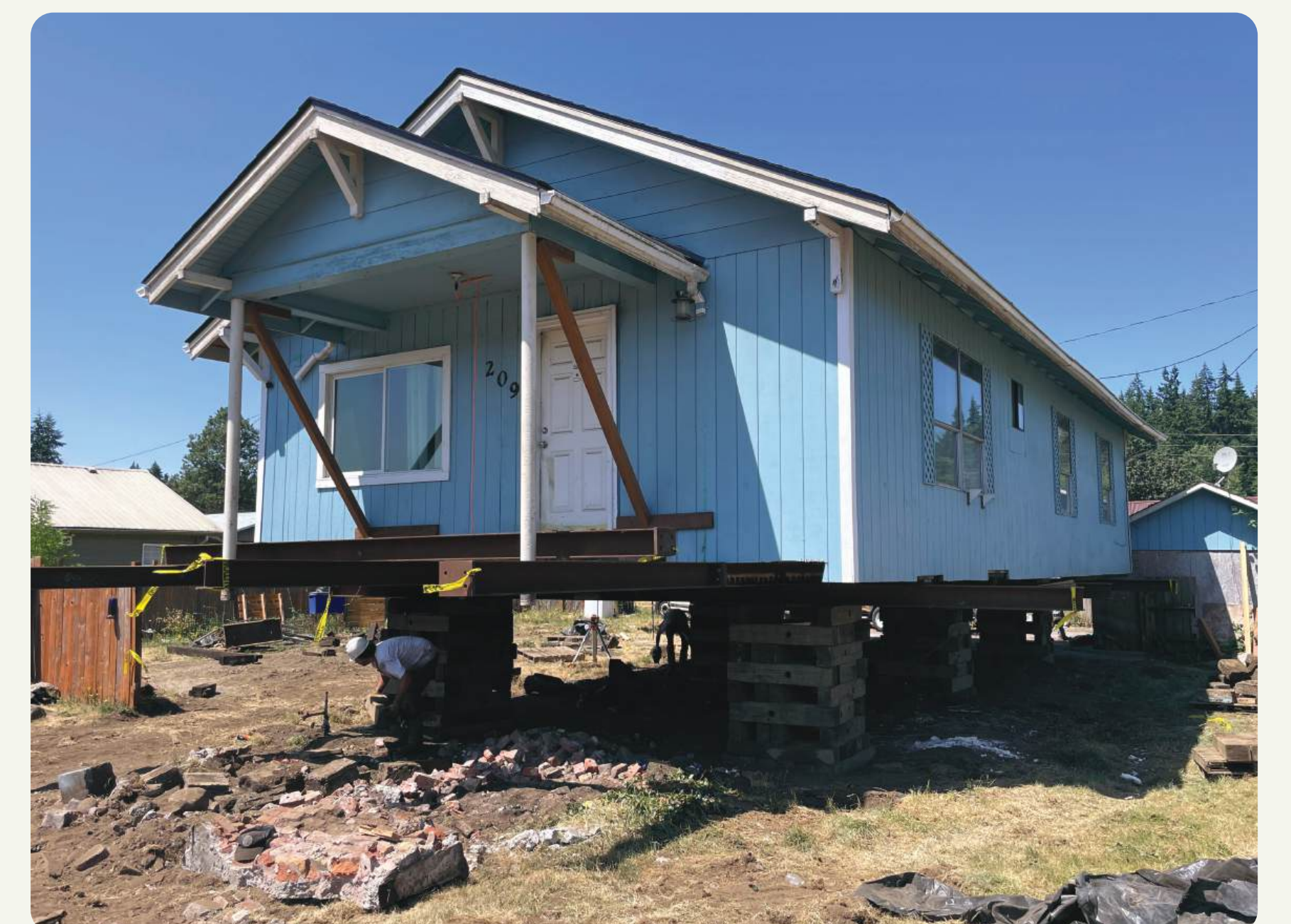
Home elevation in progress
