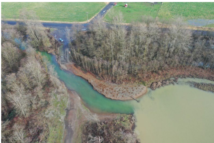
Figure 4. January 2021 drone flight showing Phase 2 restoration activities to enhance hydraulic connection and overflow channel into Pond C fully engaged.
