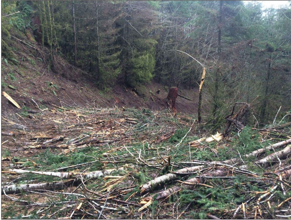
Photograph 3.1 Corduroy Road Surface for Borehole Location Access
