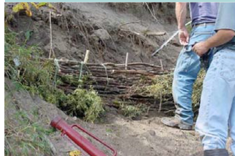
Brush Layering - Excavation of brush bench and cutting placement.
