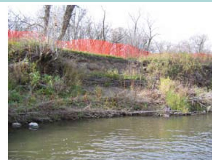
Brush Layering - Excavation of brush bench and cutting placement.
